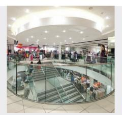
Clothes retailer New Look opted for a curved Crystal balustrade in their atrium, a Crystal balustrade with stainless steel handrail on the steps and staircase and an Onyx handrail fixed to the walls of a second staircase. Mirror-polished Onyx handrails were used throughout. We also manufactured the stairs.
